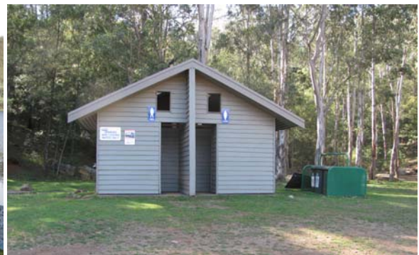
Main camping area toilet block
