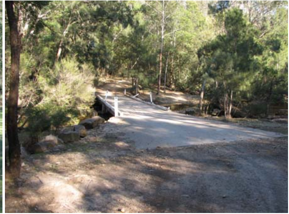
Existing bridge over Yarramunmun Creek
